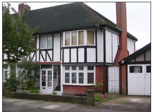
Detrimental glass front porches, pvc-U windows and inappropriate garden doors compromise the homogeneity
